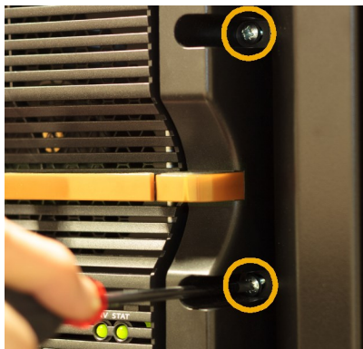
Figure 3-2: Bolting the enclosure in place, top and bottom
