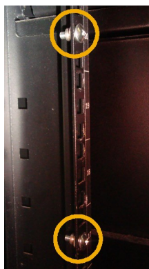
Figure 2-12: Attaching the rear rack nuts
