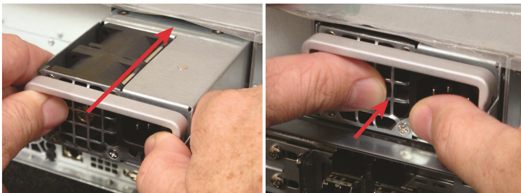
Figure 1-32: Installing the new PSU
