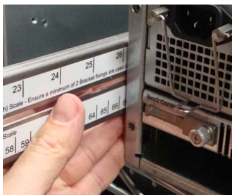
Figure 2.9: Positioning the mounting rails
