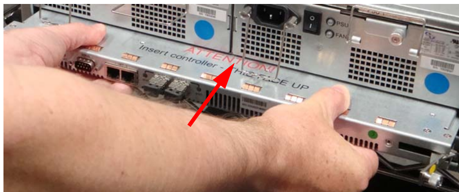
Figure 3.7: Sliding the RAID Controller into place
