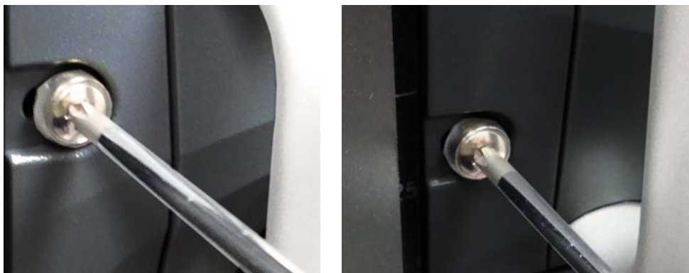
Figure 4.8: Unbolting the SATABeast/SASBeast from the rack
